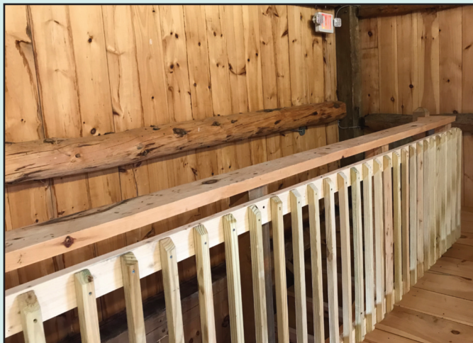
Carmine Centrella and his brother-in-law Tom Brennan built two wooden stair bannisters to required life safety code.
